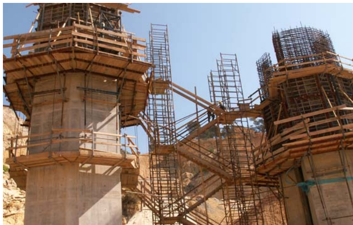
Piers under construction
