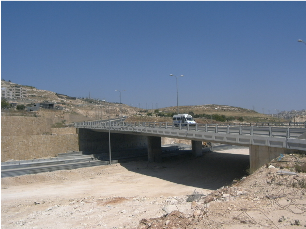
Voided slab bridge
